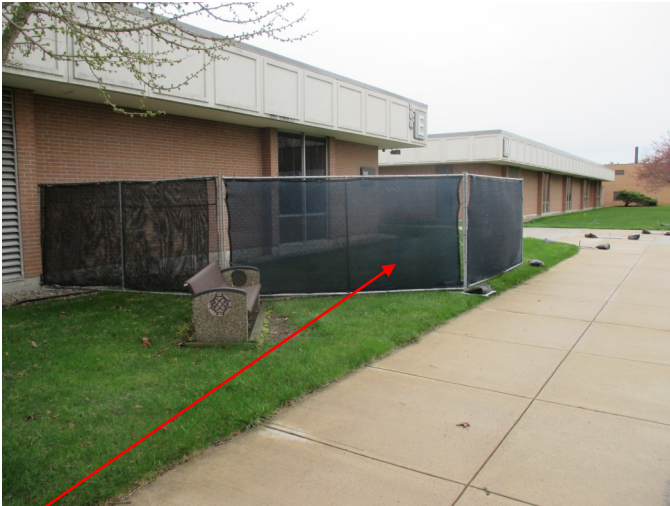
The top-left photo shows the beginning of the temporary fencing going up around the construction site. This fencing will help to contain work zones and keep pedestrians on campus safe.
